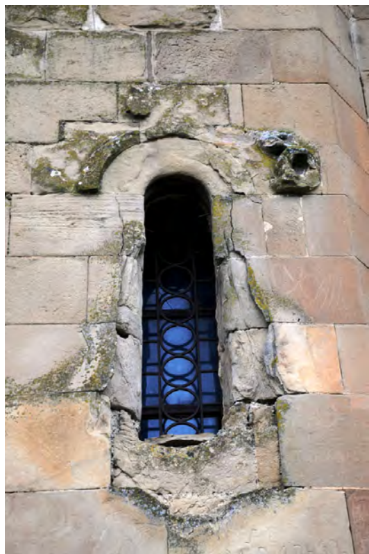
39,40. Jvari church – Great Church – Existing condition of the building blocks
