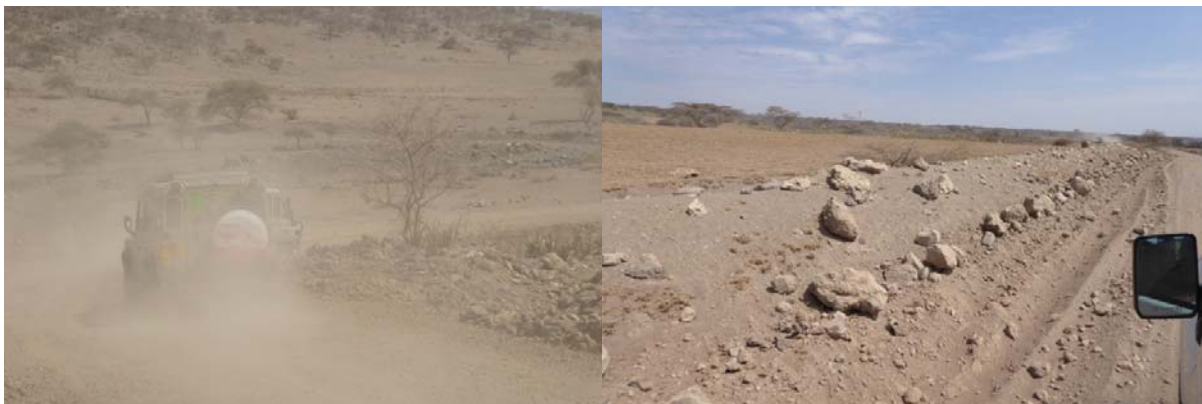
Present condition of the unsurfaced murram/gravel road through the NCA. Dusty travelling conditions (Photo 5, left) and unsightly waste material along the road verge (Photo 6, right). ©IUCN/Peter Howard.
